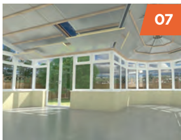
07 3 layers of high performance insulation (between and over rafters, and insulated plasterboard), is installed.
